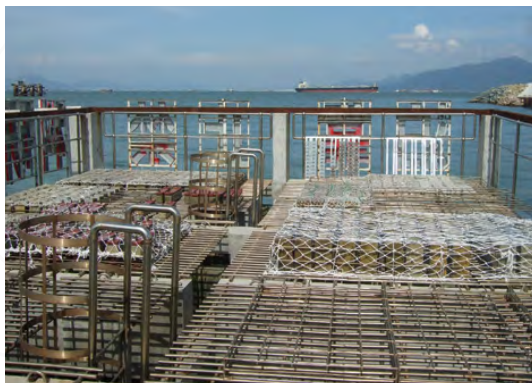
▲ Exposure site in Hongkong-Zhuahai-Macau project site, China (2013). Courtesy of HZMBA.
