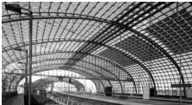
Figure 12 : voûtes bidimensionnelles. Figure 12: bi-dimensional vaults.
