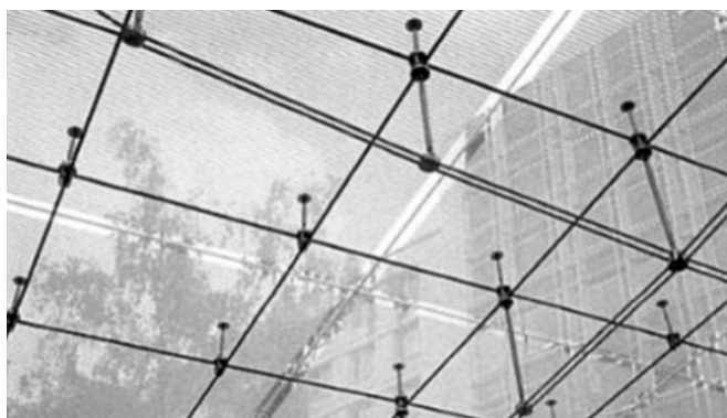
Figure 16 : nappe de câbles. Figure 16: glass walls.
