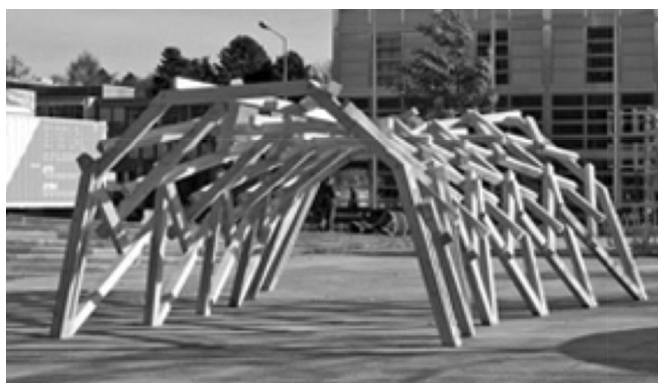
Figure 17 : nexorades. Figure 17: nexorades.
