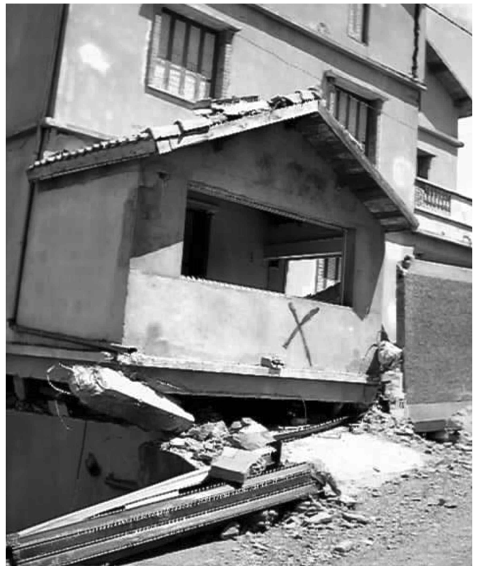
Elevation irregularity.
