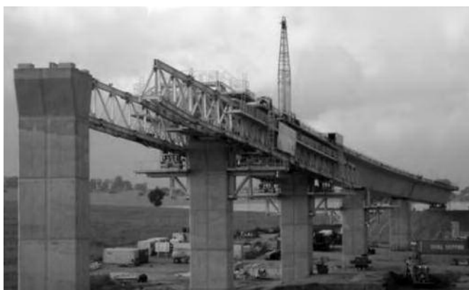
Photo 10 : Lanceur type T1/ Launcher T1.
