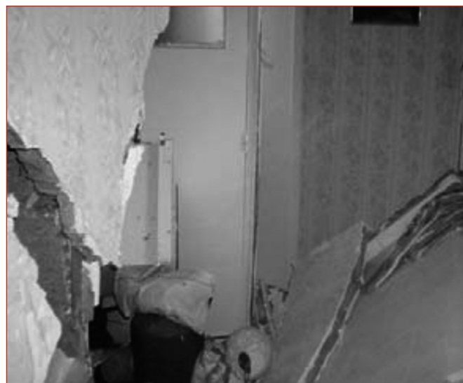
Figure 12: Effondrement et fissuration des cloisons.
