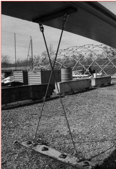
Figure 13 : Appui central croisé.
