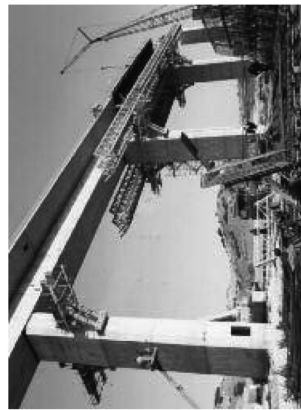
Underslung traveller for span-by-span construction process (movable shuttering system), Anchuelo Viaduct high-speed railway Madrid-Barcelona (Spain).
