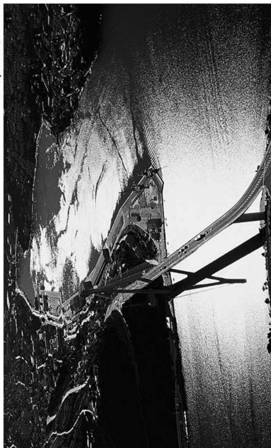
Dubrovnik bridge – single pylon cable stayed bridge
