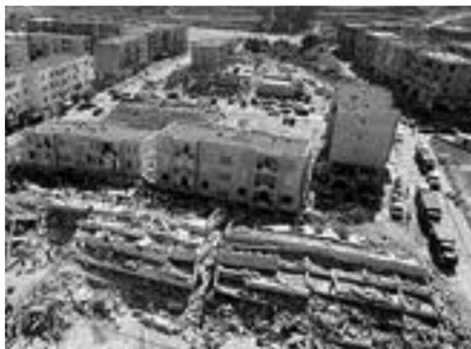
RC buildings damaged by recent earthquakes Ain Temouchenet 1999 and Boumerdes 2003.
