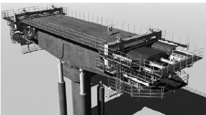
Photo 12 : Equipage mobile / Form traveller.
