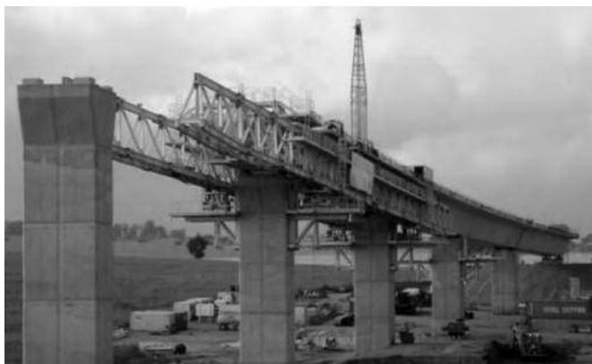
Photo 10 : Lanceur type T1/ Launcher T1.
