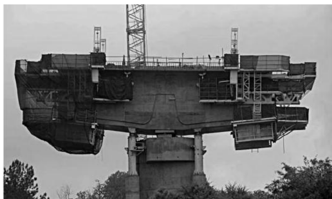
Photo 12 : Equipage mobile / Form traveller.
