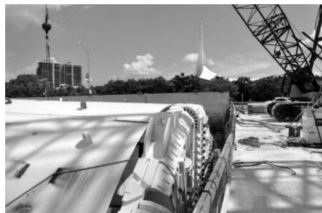
Fig 6. TBM in launching shaft
