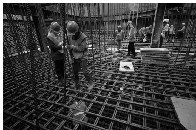
Figure 3 : Reinforcement work of MahaNakhon mat foundation/aciers du radier (Source PACE Development PLC)
